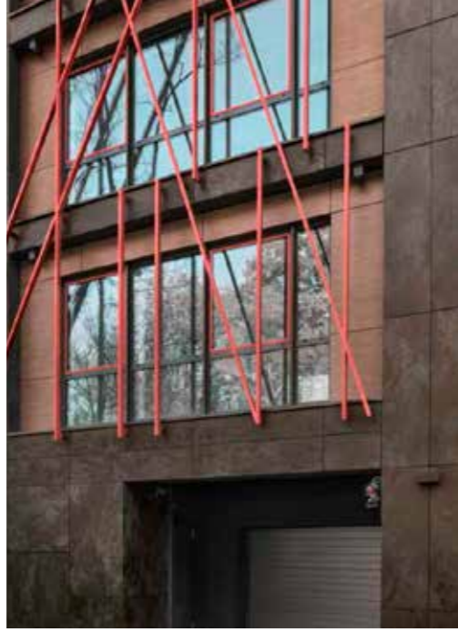
/ Warszawa Year: 2014 Portico Office Building Warszawa / Poland Laminam 3+ Ventilated Facades Oxide Nero 1000x3000 >
