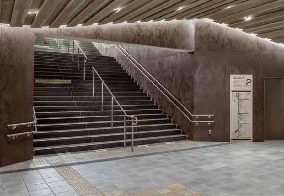
/ Tokyo Year: 2015 Takaosanguchi Station Tokio / Japan Design: Kengo Kuma and Associates + Keio Construction Laminam 3+ Oxide Moro 1000x3000 <
